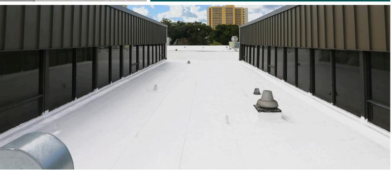
Joseph Caleb Daycare, an early childhood education center in Miami, received a new selfadhered, modified bitumen roof system installed by Florida Building & Supply. The three-ply system was built with Elastoflex SA V for base and interply sheets, and Polyfresko G SA highly reflective white cap sheet. This system features Polyglass' CURE Technology®, which provided the required energy ratings; and ADESO® Technology, which allowed the daycare center to remain open during the roofing project.
