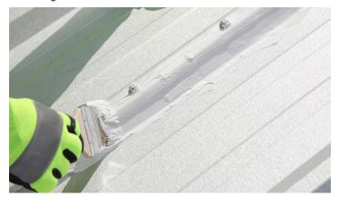
At the interface of any metal with a dissimilar material, detail the joint using one of the following methods:
