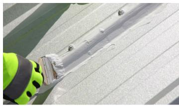
At the interface of any metal with a dissimilar material, detail the joint using one of the following methods:
