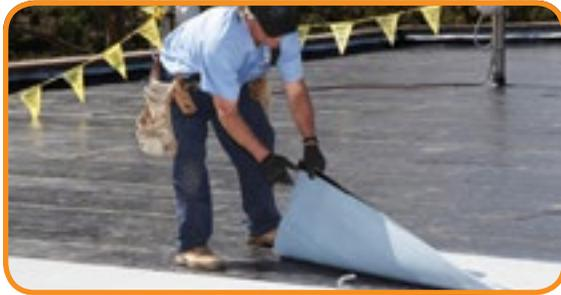
Lay the membrane on the roof aligned with the eaves edge at the lowest point on the roof.
