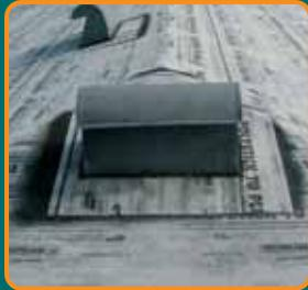
1. Application of an overflow detail.
