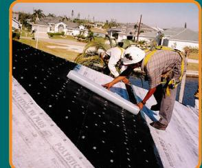
**1.** All applicable substrates should be dry, clean and properly prepared before any application of Polystick underlayment.
