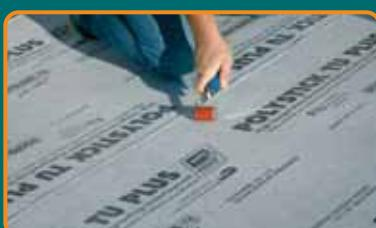
**4.** Selvage area must be rolled with a hand roller to ensure full contact to the substrate.
