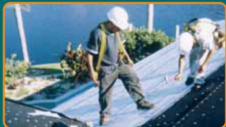
**3.** All rolls should be back-nailed in the selvage area as per POLYGLASS' back nailing guide. The POLYGLASS® nailing pattern requires that fasteners be centered within the 3" selvage and placed 12" O.C. The fastening shall be through the top fabric surface and the membrane into the acceptable substrate. Fasteners must be 11 gauge, ring-shank type, and applied with minimum 1" tin disk. (Refer to the **POLYSTICK TU PLUS** installation detail).
